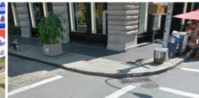
Missing Curb Ramp
